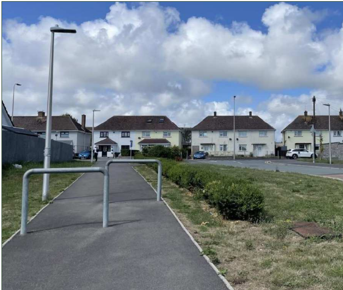
Photograph 2.3 – Rhoose Way Cycle / Footway
